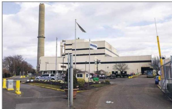
Covanta operates four waste-to-energy plants on Long Island, including this Westbury facility. It owns three out of the four plants.
